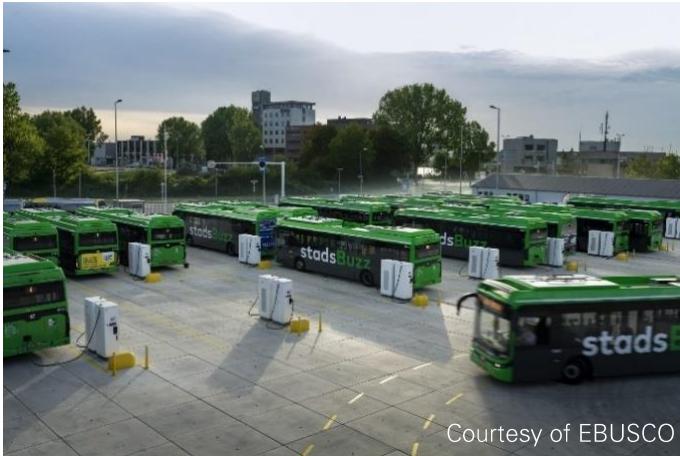
Figure 9. Modern Bus-Depot with Charging Infrastructure
